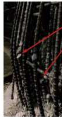
Damage due to insufficient splices
